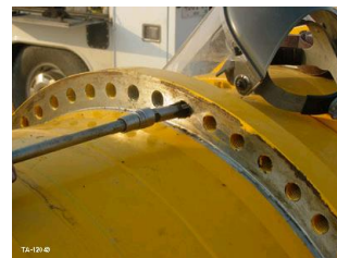
Cleaning paint and rust prior to torquing
